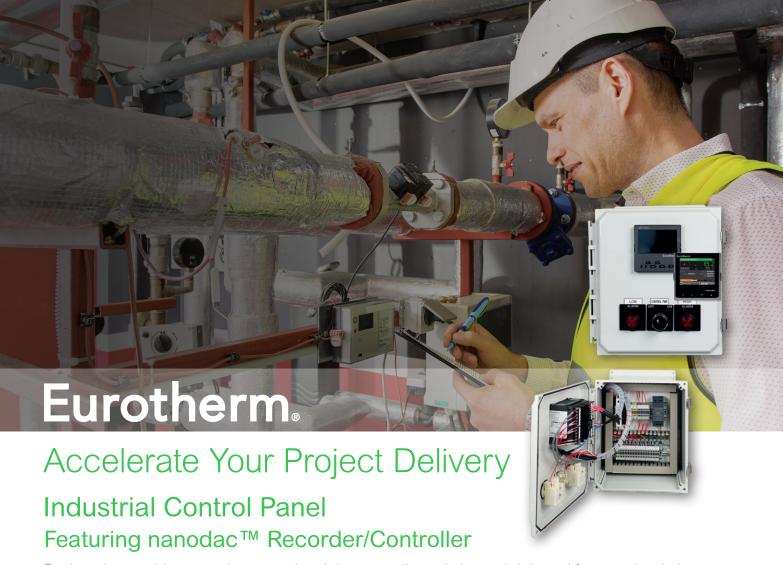
Designed to provide a complete control and data recording solution and delivered from stock to help meet short lead times, this industrial panel with Eurotherm nanodac recorder/controller is ideal for projects where a custom control panel has not been budgeted for and fast delivery is needed. Its standardized UL508A approved design satisfies a variety of machine control applications.
